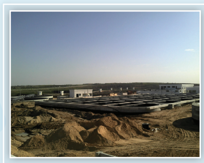
Photo 2. NGEST under construction
