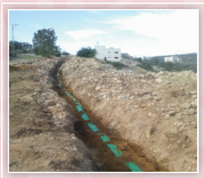
Installation of wastewater network in Barta'a Al-Shariqia
