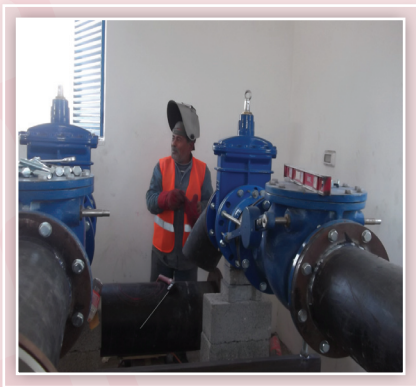
Upgrading of water supply system in Rafah
