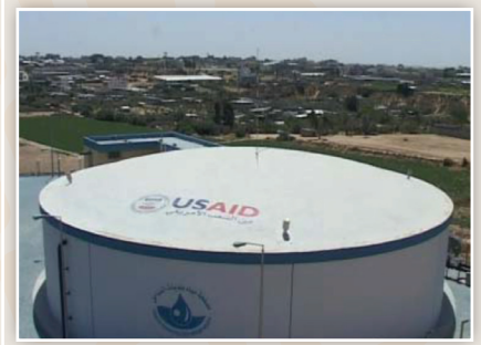
3 A 5000 meter 3 water reservoir constructed by USAID in Khan Younis to reduce the water shortage faced by area residents. The new water reservoir provides water to 70,000 people in the town.
