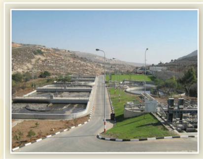
Al-Bireh WWTP commissioned in year 2000
