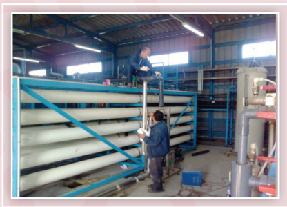
Upgrading of Deir Al-Balah Desalination plant
