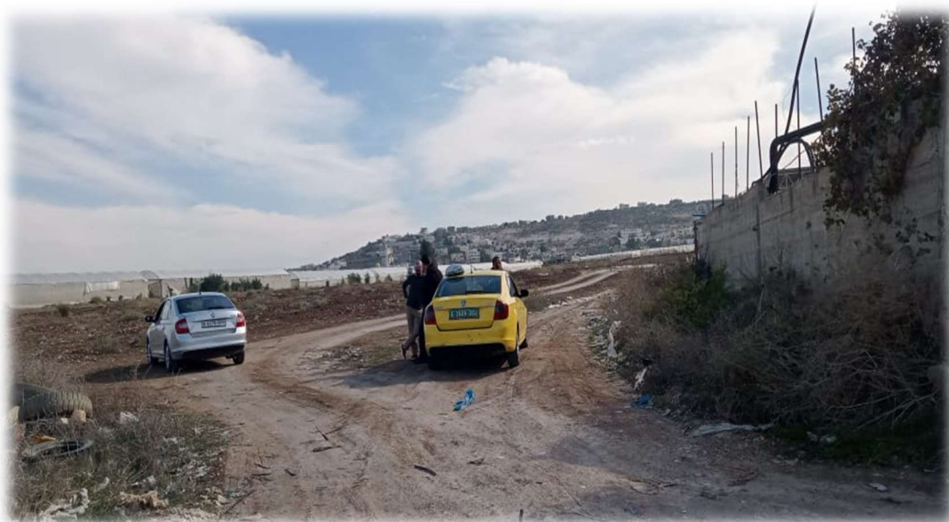
Photo for Land of Qabatiya Booster Pumping Station Adjacent to Abu Arab Well
